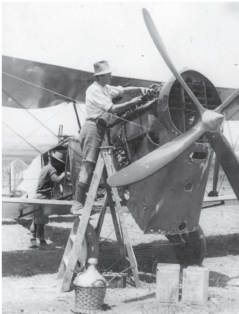
Cpl Laurie Matulich of 1 AFC works on a Bristol Fighter engine in Palestine in 1918. The propellers of the Bristols were 2- or 4-bladed depending on the version of Rolls-Royce Falcon engine fitted.
